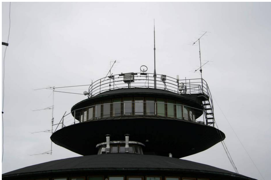
Po lewej- 4x 6el SP9FYS Yagi fixed to West with 52 deg in horizon,
